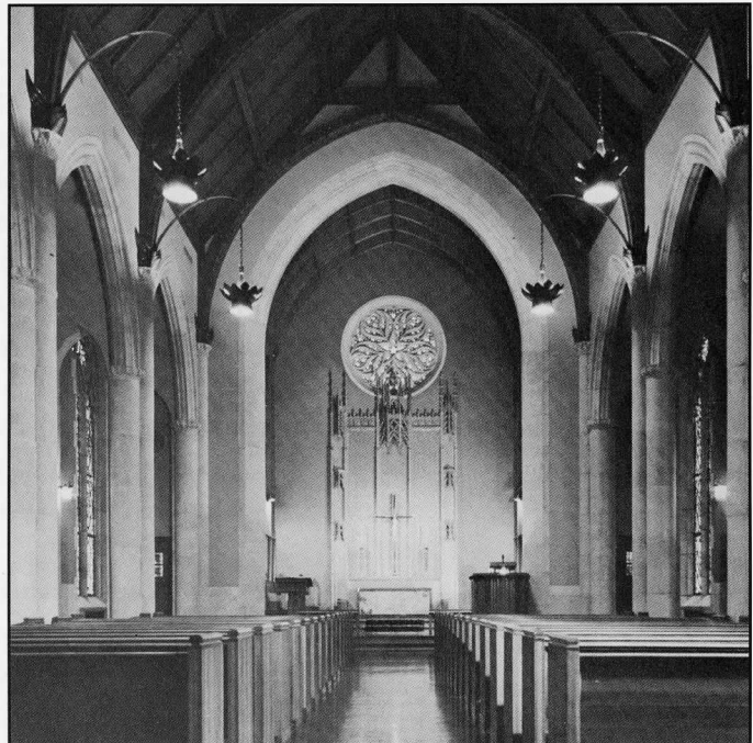
Cox Chapel interior remodeling included repainting, refinishing of the pews, improving the sound system, a new parquet floor, and renewal of the altar area.
